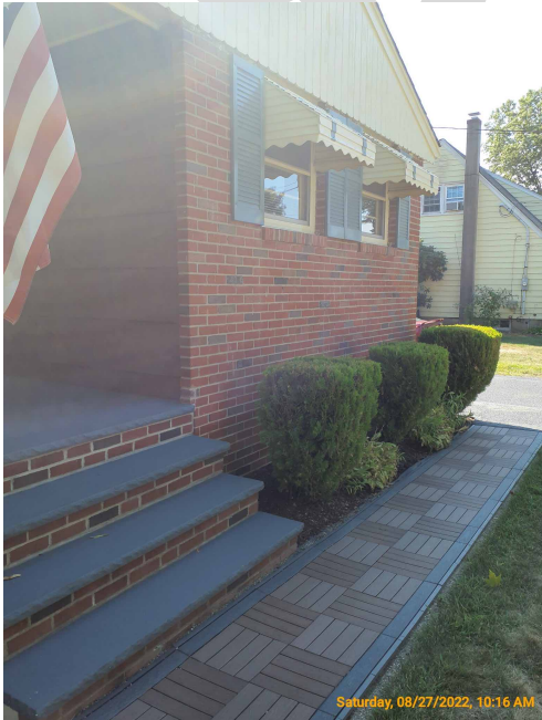
13: Secondary exterior wall covering: Brick veneer
