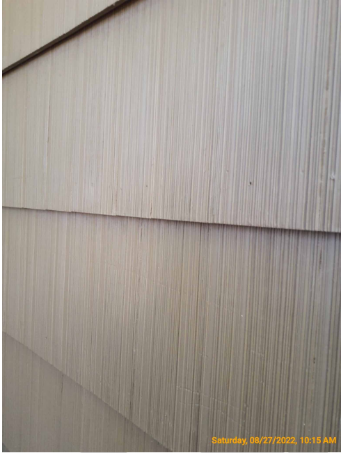
12: Primary exterior wall covering: Wood shingle siding, painted
